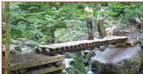
Bridge on Northville-Lake Placid Trail Reroute
