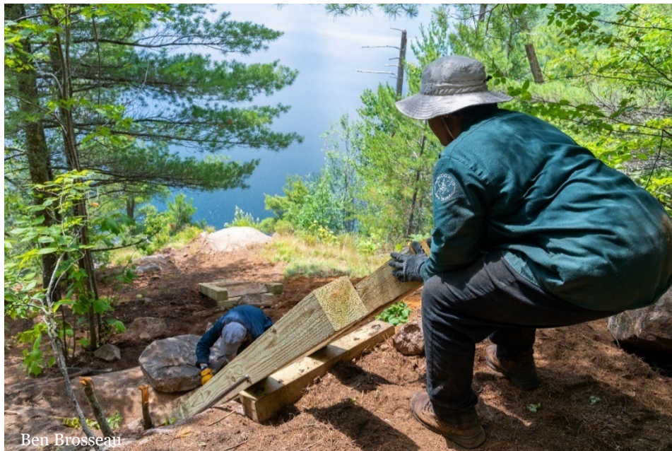
Professional trail crew members set up parts of the dimensional wood staircase to custom cut portions of the lumber for an exact fit.
