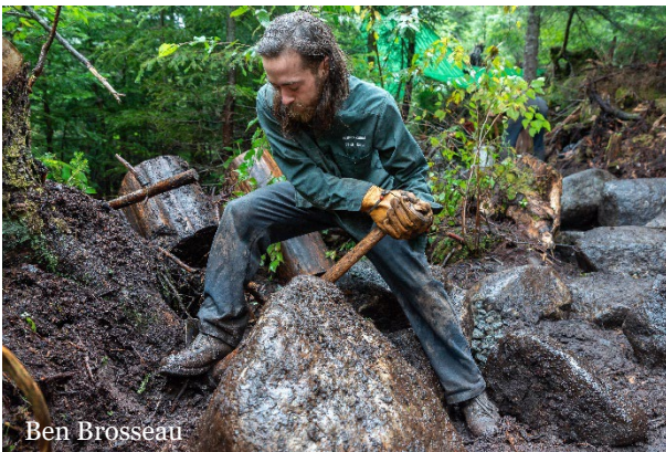
A professional trail crew member works to set a rock for turnpiking near Avalanche Lake.
