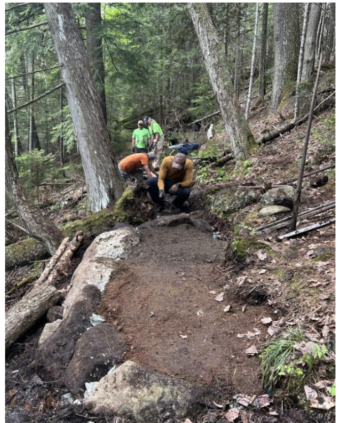
Volunteers build a rock turnpike
